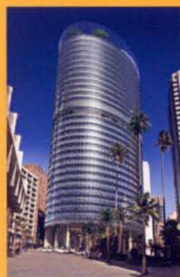
Architectus provided Urban Planning and Architecture services for 1 Bligh Street, Sydney - a 6-Star Green Star office tower co-owned by DEXUS Property Group and Cbus Property
